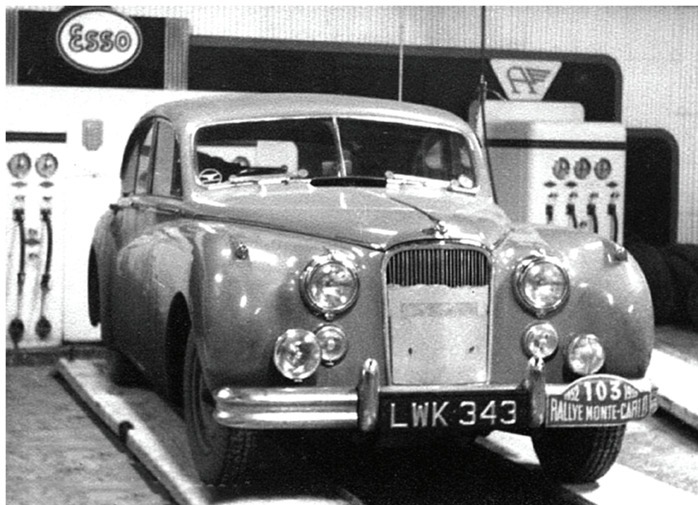
LWK 343: Mk VII Jaguar prepared for the 1952 Monte Carlo rally and fitted with a makeshift radiator blind to maintain engine temperature in the freezing conditions. This Jaguar also won at Silverstone in the same year in the hands of Stirling Moss, and was used the following year to gain a speed record (121.704mph) at Jabbeke, in Belgium, in the hands of Jaguar test driver Norman Dewis. Moss again won in this car at Silverstone in 1953, and in 1955 Mike Hawthorne led home a trio of Mk VII Jaguars to win at Silverstone in this very car.
